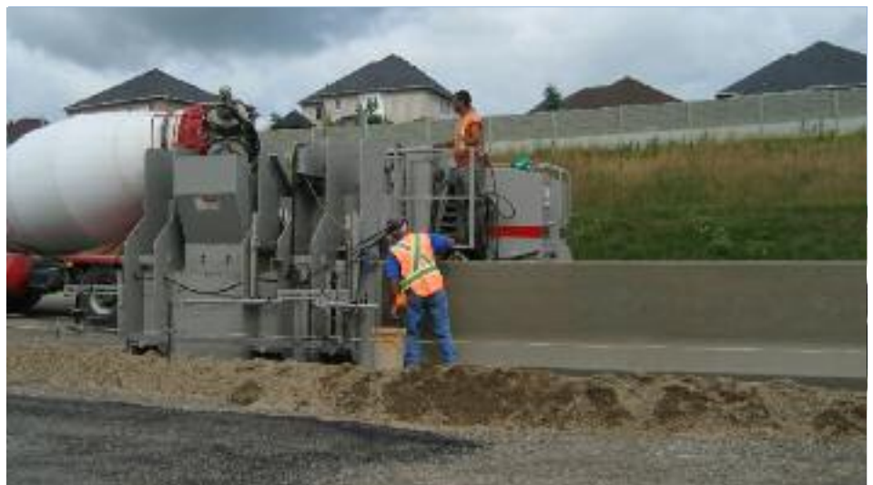
Variable barrier, up to 68" (1.72m) tall.
