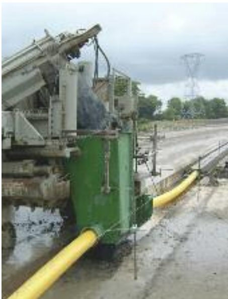
Slotted drain in Uzbekistan showing inflated tube.
