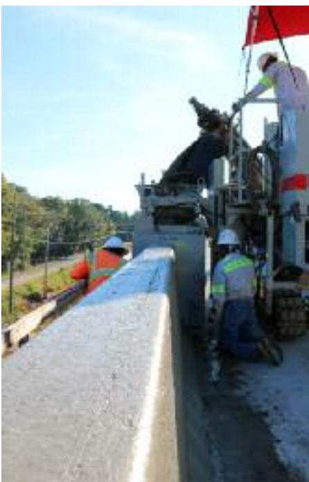
Close up of Bridge Parapet
