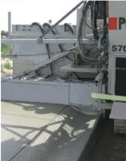
Monolithic curb, gutter, and sidewalk.
