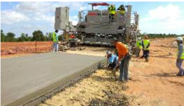
▲ Power Curbers 7700 Multipurpose Slipform Machine Paving
