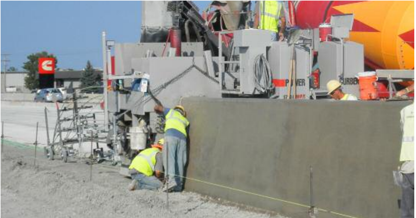
Variable barrier pour from 58" to 70" (1.47 - 1.78m) tall.
