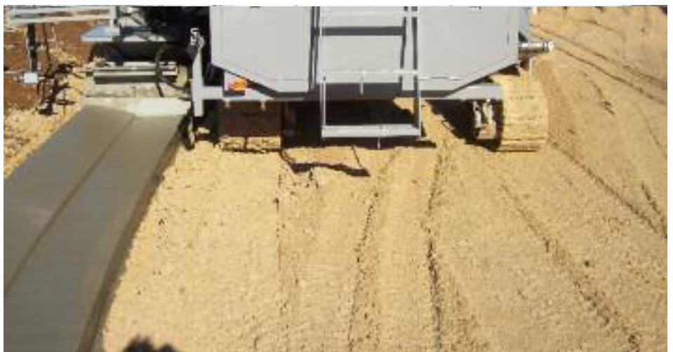
The machine handles muddy and rough conditions.
