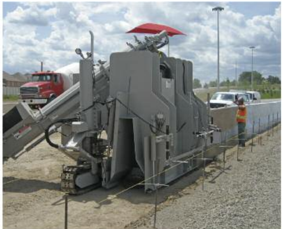
MAX package pouring large variable barrier wall.
