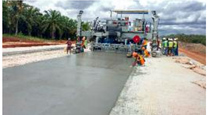
▲ Power Pavers Full-Sized, 4-Track SF-2404 Slipform Paver
