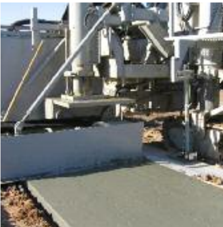
Sidewalk adjacent to back-of-curb. Sensing off-curb.
