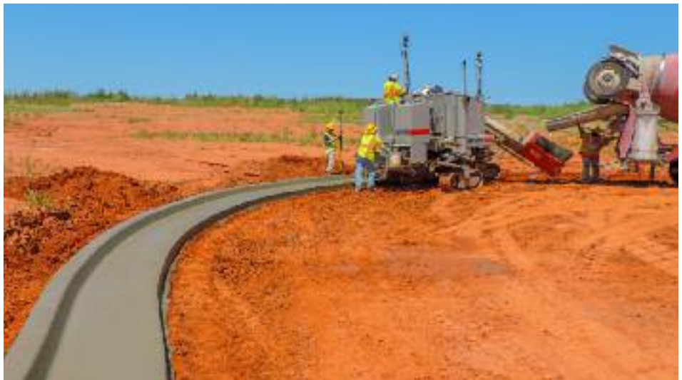
The 5700-D is fully stringless capable
