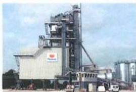
300 tonne horizontal Hot Storage
