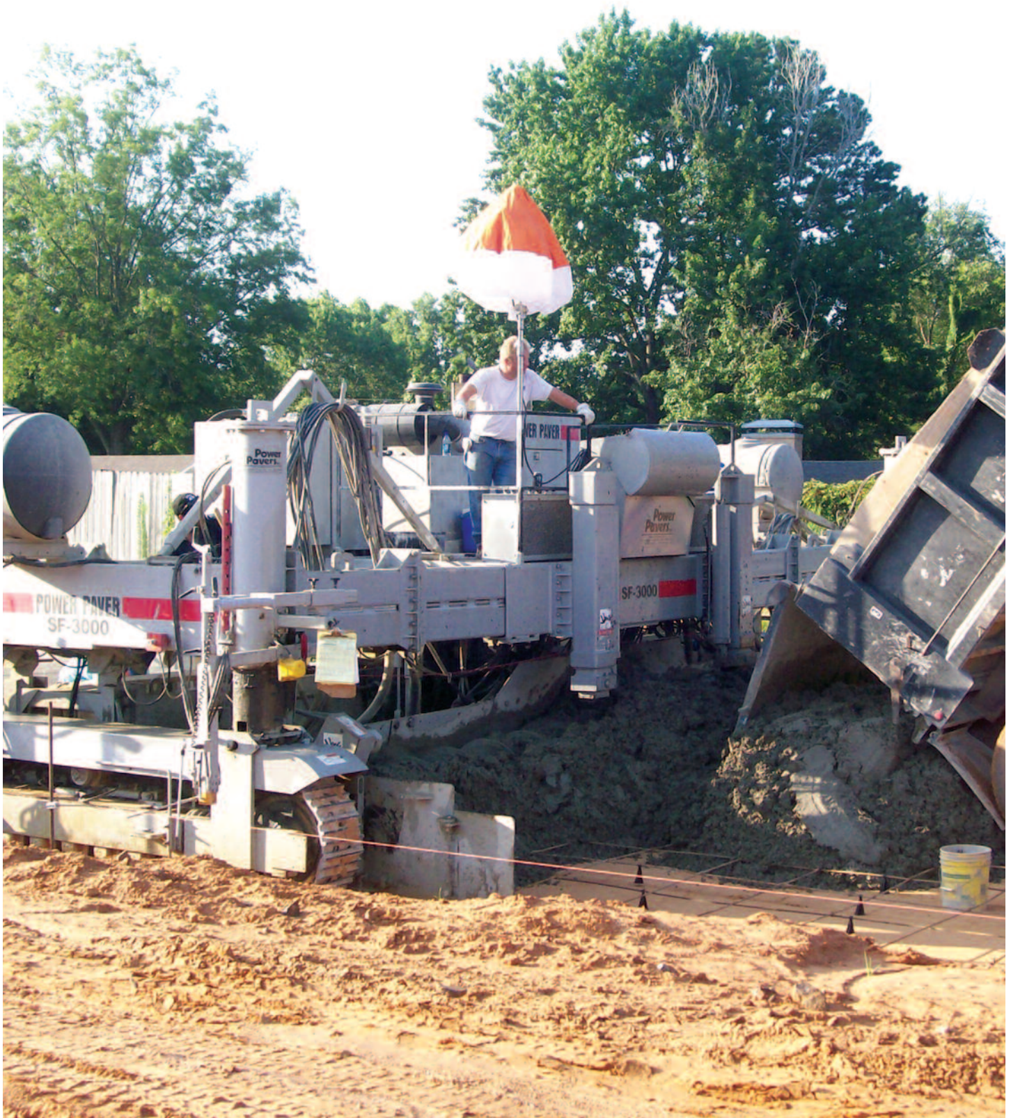
SF-3000 has the size and power to handle large volumes of concrete. Here it is paving over steel reinforcement.
