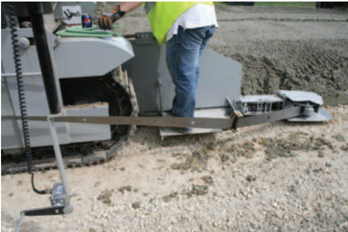
Optional key-way inserter with manually placed tie bars.
