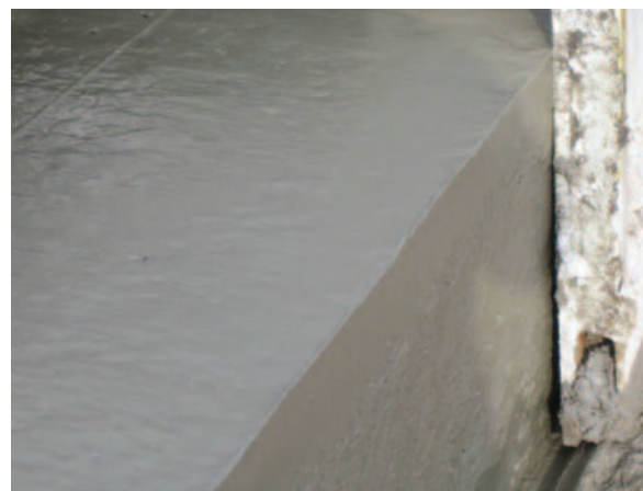
Everything works together to create pavement with smooth flat finish and a sharp square edge.
