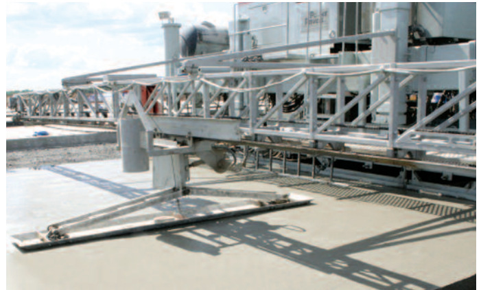
Optional final finisher features an oscillating mechanical float.
